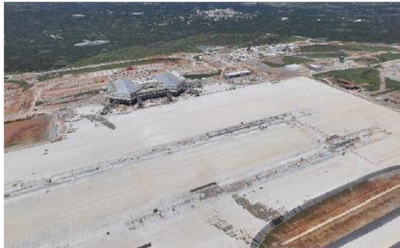
Apron Pavement Works
