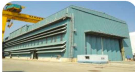
Approx 3,000 sq. m. PEB installation with a retractable (openable) roof structure for a Kolkata based shipyard
