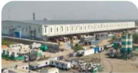
Over 57,000 sq. m. PEB installation for a warehouse, for a multinational e-commerce company at Ahmedabad, Gujarat
