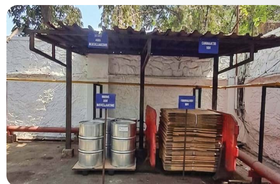
■ Waste Segregation at Turbhe Site
