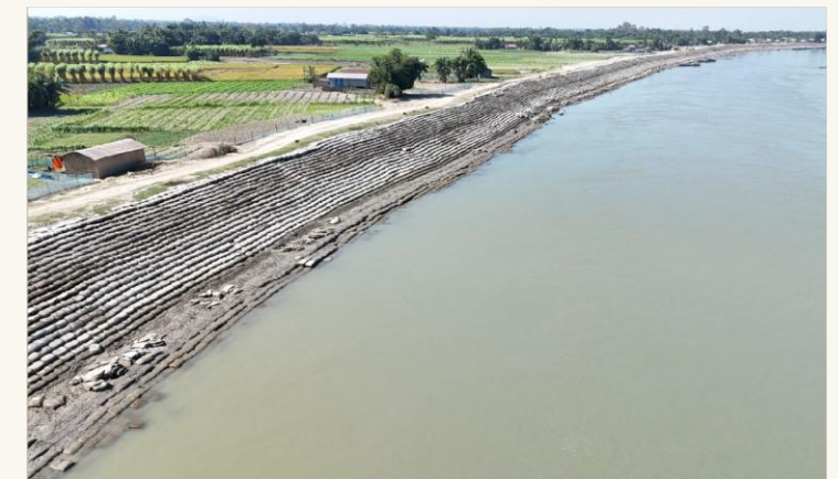
P1 & P2 Riverbank Protection, Palasbari, Assam Completed
