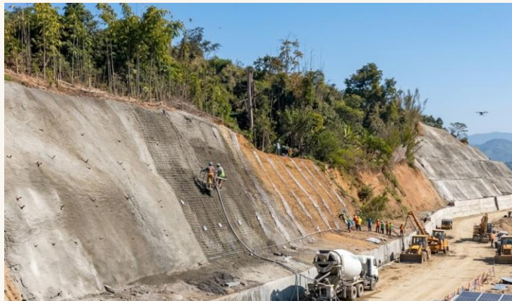
Slope Protection (Hilly Areas), Mizoram Completed
