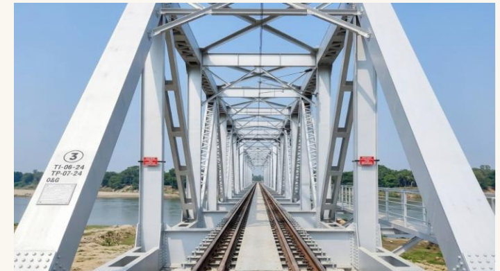
Rangia Bridge, Assam North east · Completed
