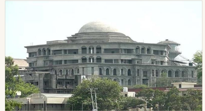
Legislative Complex, Jammu Ongoing
