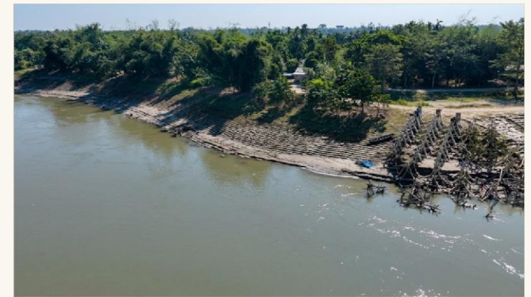
Riverbank Protection, Lakhimpur, Assam Ongoing
