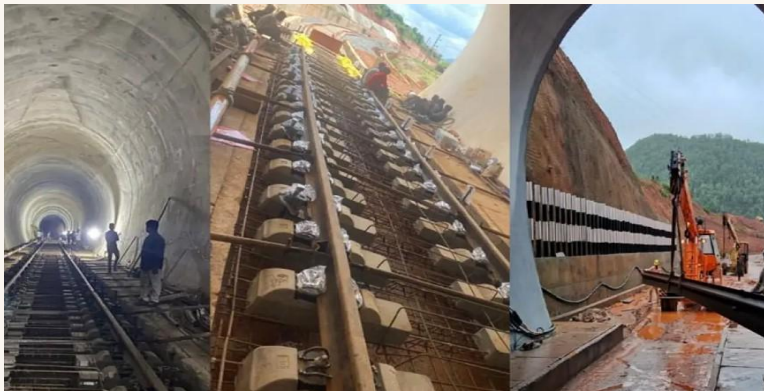
Six Tunnels, Boddavara, Odisha North east- Ongoing
