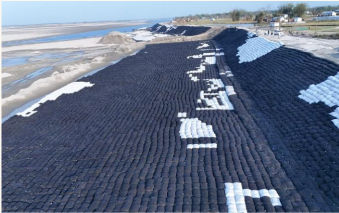
PGA Anti-Erosion Works Ongoing
