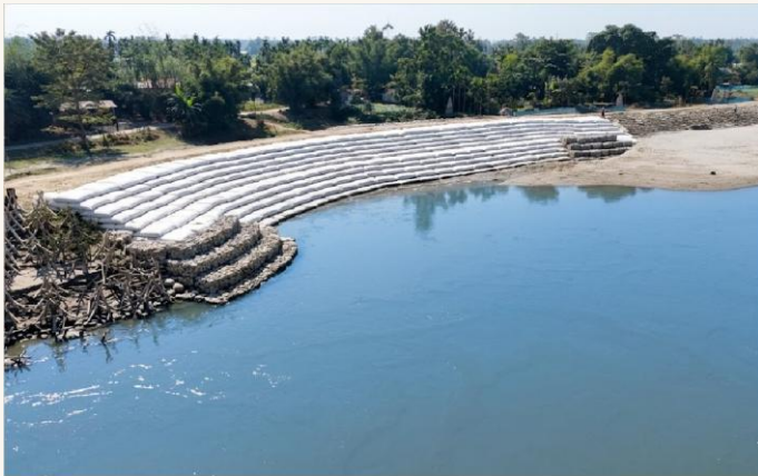
Riverbank Protection, Dibrugarh, Assam Ongoing
