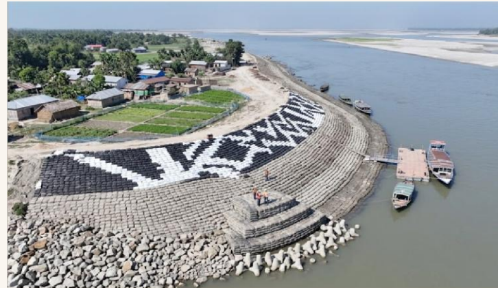
Golaghat & Sibsagar Anti-Erosion Works, Assam Ongoing
