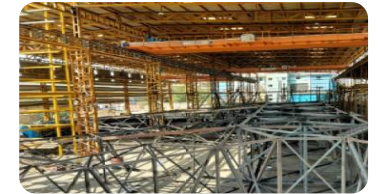
TLT & Wind Angular Tower, Tarapur
