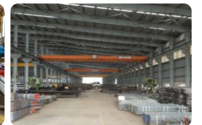
Solar Piles & TLT, Bhachau, Gujarat
