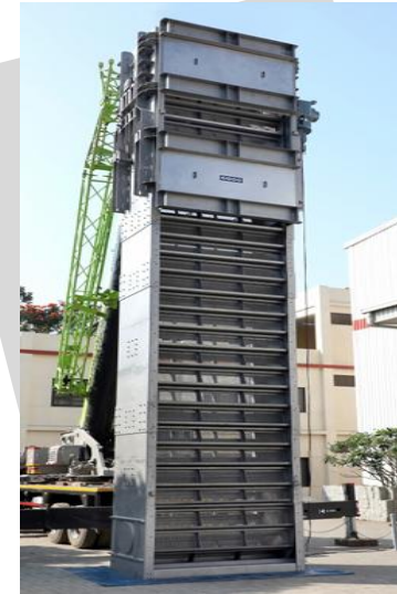
Bangkhen Water Treatment Plant in Bangkok, Thailand
