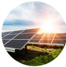
Solar EPC Projects
